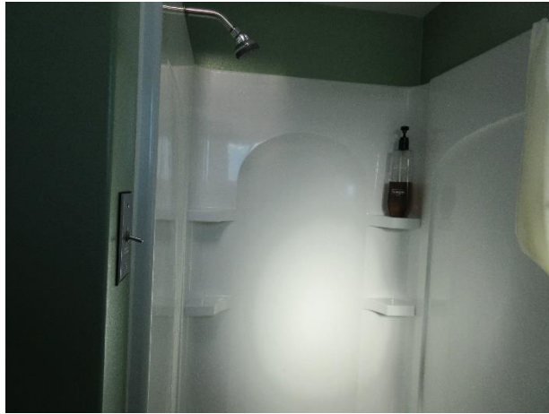
Guest shower stall with wall switch for pump
